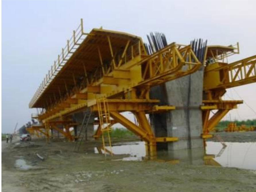
**Figure 6-3: Example of Travelling Shoring System**
