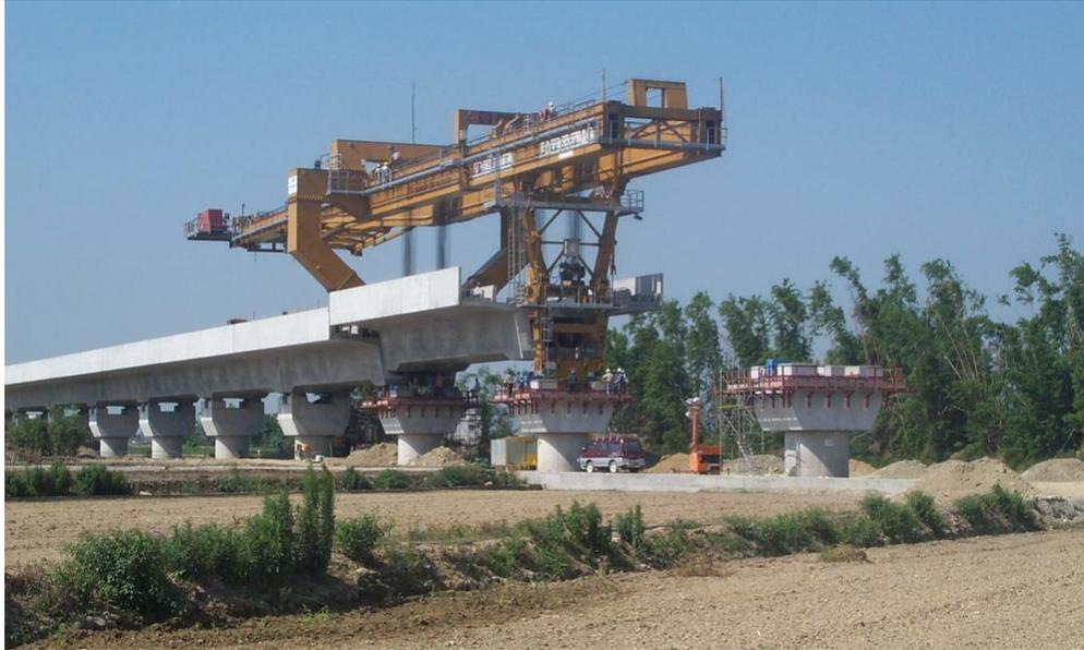
**Figure 3-13: Example of Overhead Gantry**
