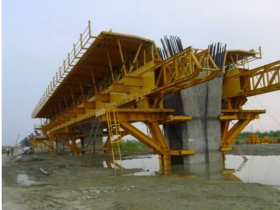
Figure 6-3: Example of Travelling Shoring System
